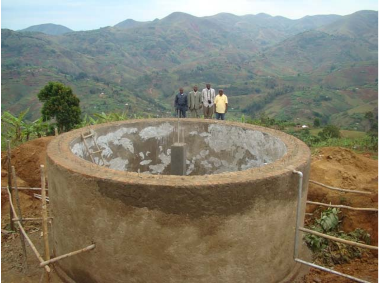
Banro Foundation staff with the tank for a potable water system near the Twangiza gold mine project in the eastern DRC. It serves 18,000 people and consists of 19,000 metres of piping.
