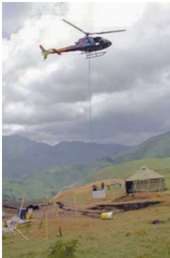
Helicopter support is essential to the core drilling
